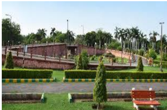
(c) Traffic Park front view
