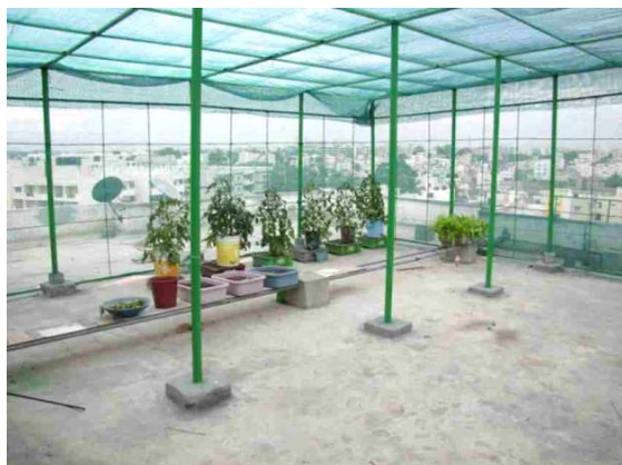
(c) Green roof at a house
