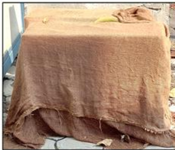
Fig. 5. Curing of panel
