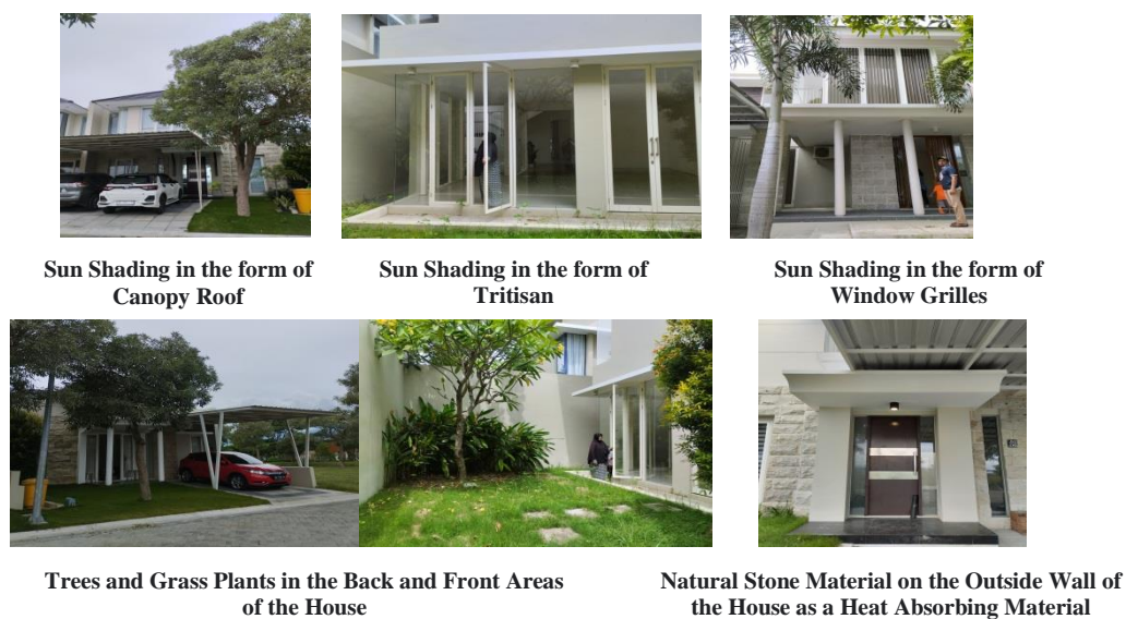
Fig. 1. Bioclimatic Architecture Strategy to Anticipate Solar Thermal Radiation at Citraland Residential Houses
